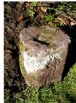
A socketed mullion section of window stone made of Old Red Sandstone from Turriff.
